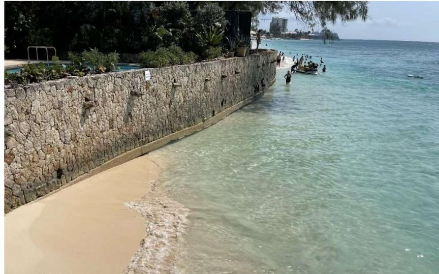
**Figure 5-2 Vertical wall at the beach directly exposed to waves do increase beach erosion due to the effect of wave reflection from the wall. Photo: DHI**
